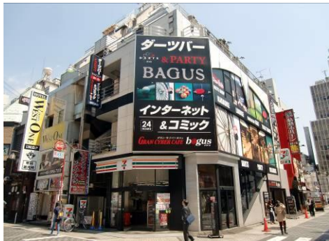
Nishi-Ikebukuro 1 Chome Building
