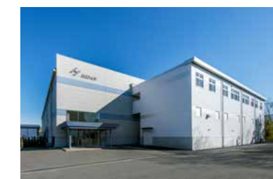
Funabashi Hi-Tech Park Factory I
