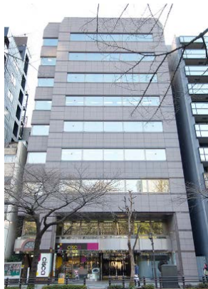
Hiei Kudan Building
