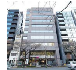
Hiei Kudan Building
