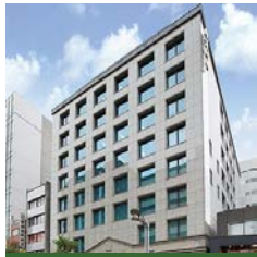
OF-01 Seishin Bldg
