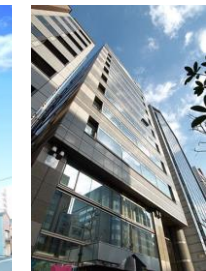
NK BLDG. (Chiyoda-ku, Tokyo)
