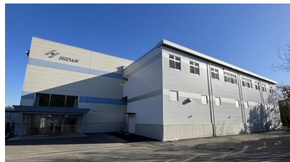
The right side of the photograph shows one of the 2 spots where the building was extended.
